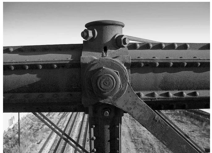
Figure 1. Upper chord pin-and-eyebars connection in an 1881 Whipple Phoenix Truss. The eyebars and compression sections are wrought iron, the joint blocks are gray cast iron, and the pins are wrought iron on the upper chord and steel on the lower chord.
